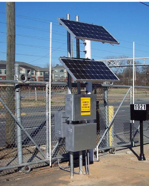
**Solar panels can power electric fence systems, ensuring a disruption to the power supply will not leave a facility vulnerable to theft.**
